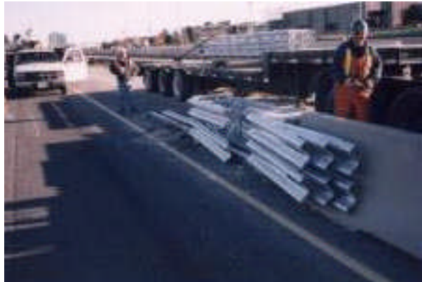
TRACC Replacement in Progress
