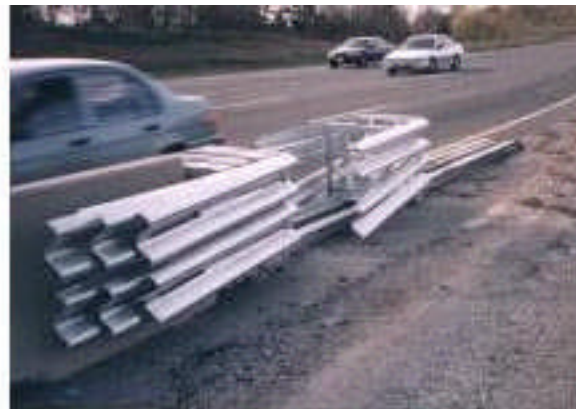
Damaged TRACC Prior to Replacement
