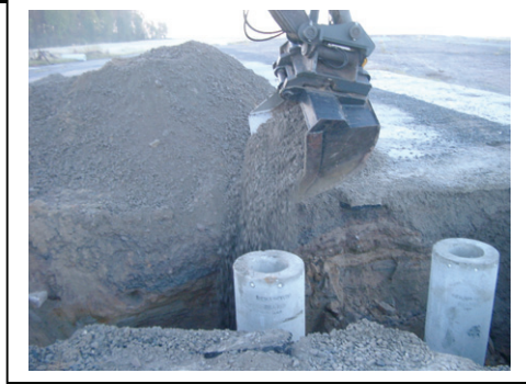
Install foundation & backfill
