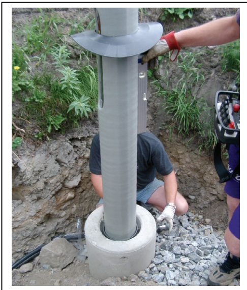
Locate post in foundation and level. Tighten Fixing Bolts onto Compression Ring
