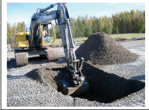
Excavate trench or hole
