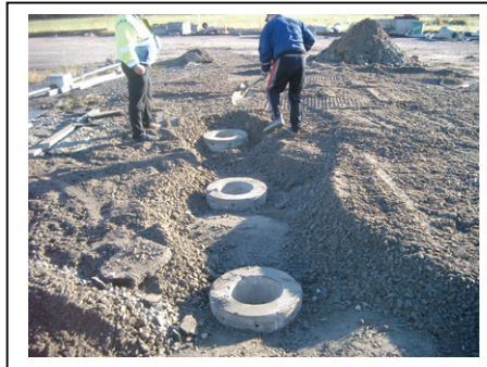
Backfill to within 100mm from top
