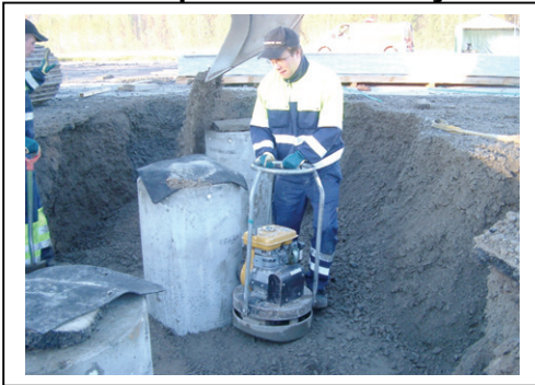
Compact backfill in layers
